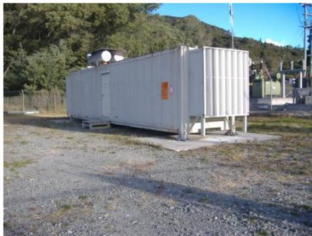
ENL purchased 6 x 1.25MVA Diesel Generators in 2002 that supply at 11kV and include TOU metering. The units are capable of being relocated as required.
