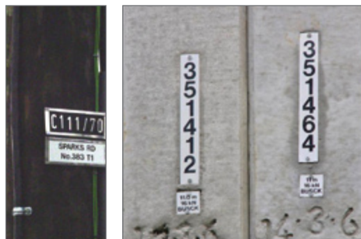
Photo 2: Many electricity network poles carry some form of identification number. From this the electricity network company can usually tell the pole location.
