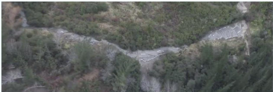
Figure 2.3: Road loss at Tauwhareparae due to major earth movement
