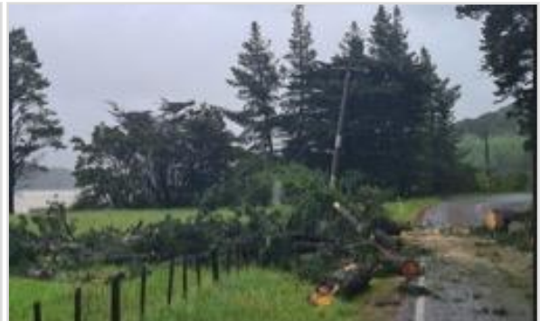
Figure 48: Line damage caused by forestry trees outside the fall zone in June 2022
